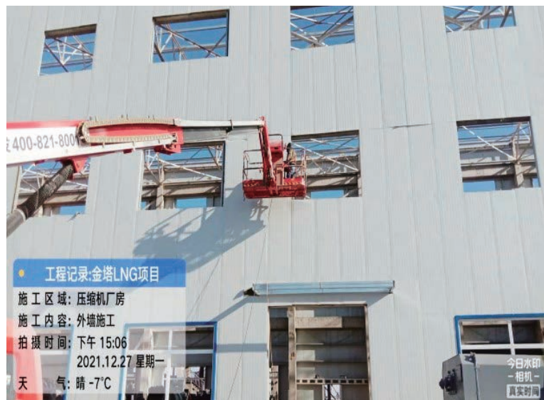
Aerial Work Picture of Xindi Energy
